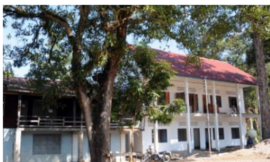
The new TMPL infants' facility at the Deak Kum Pa School & Orphanage in Luang Prabang, Laos.
